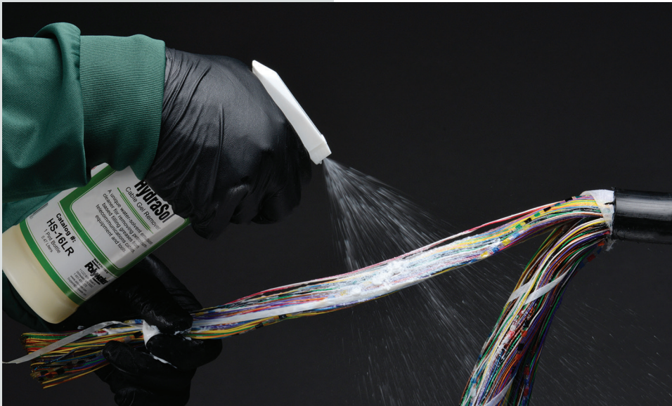
Prepping copper cable for cleaning icky-pic
