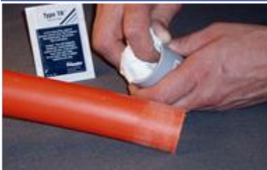
Clean Coupling and Conduit with Cleaning Wipe
