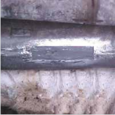
“PILC” lead cable repair
