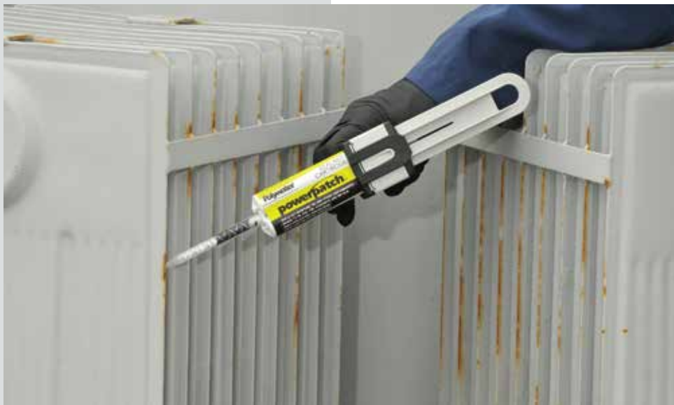
Transformer radiator fin repair
