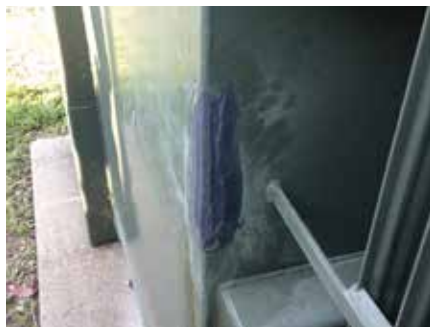
Pad-mounted transformer repair
