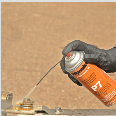
Loosening pole line bolts
