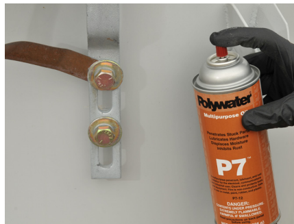
Liberally apply P7 to loosen
