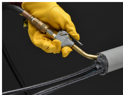
Blowing CableFree through conduits
