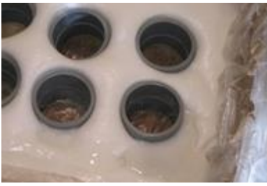
Finish installing InstaGrout
