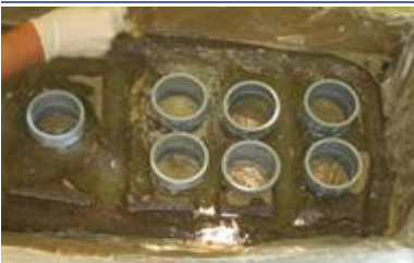
Spread the InstaGrout with a stick
